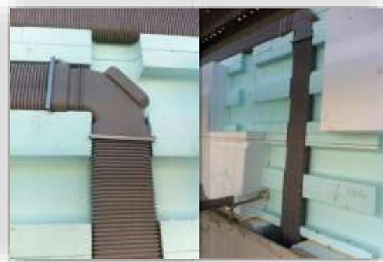
Figure 15 Façade insulations systems including air ducts
